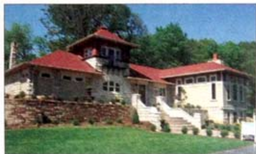
The Frisco Train Depot was restored in 2006.
